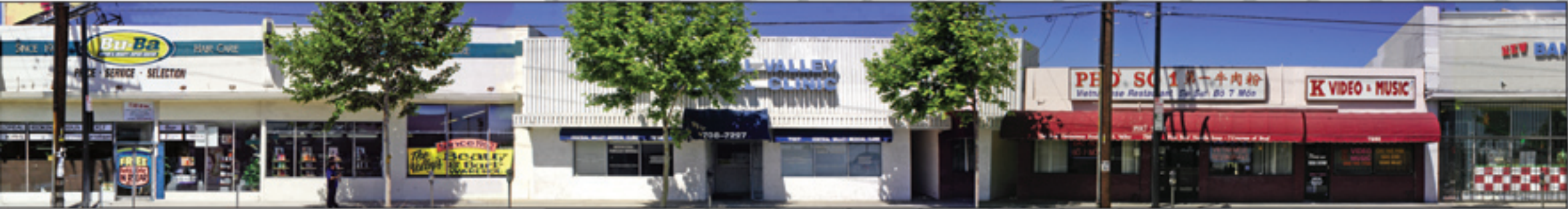
RESEDA FAÇADE AND SIGNAGE IMPROVEMENT PROGRAM: EXISTING
